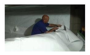
**7f** Tape any open seams at the front opening of the crawl space and install final trim piece on the opening.
