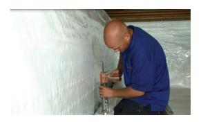
**7c** Tape all seams and around piers using the seam tape. NOTE: Try to get the liner and tape to be parallel to the ground. This is purely cosmetic, but makes for a cleaner finish.
